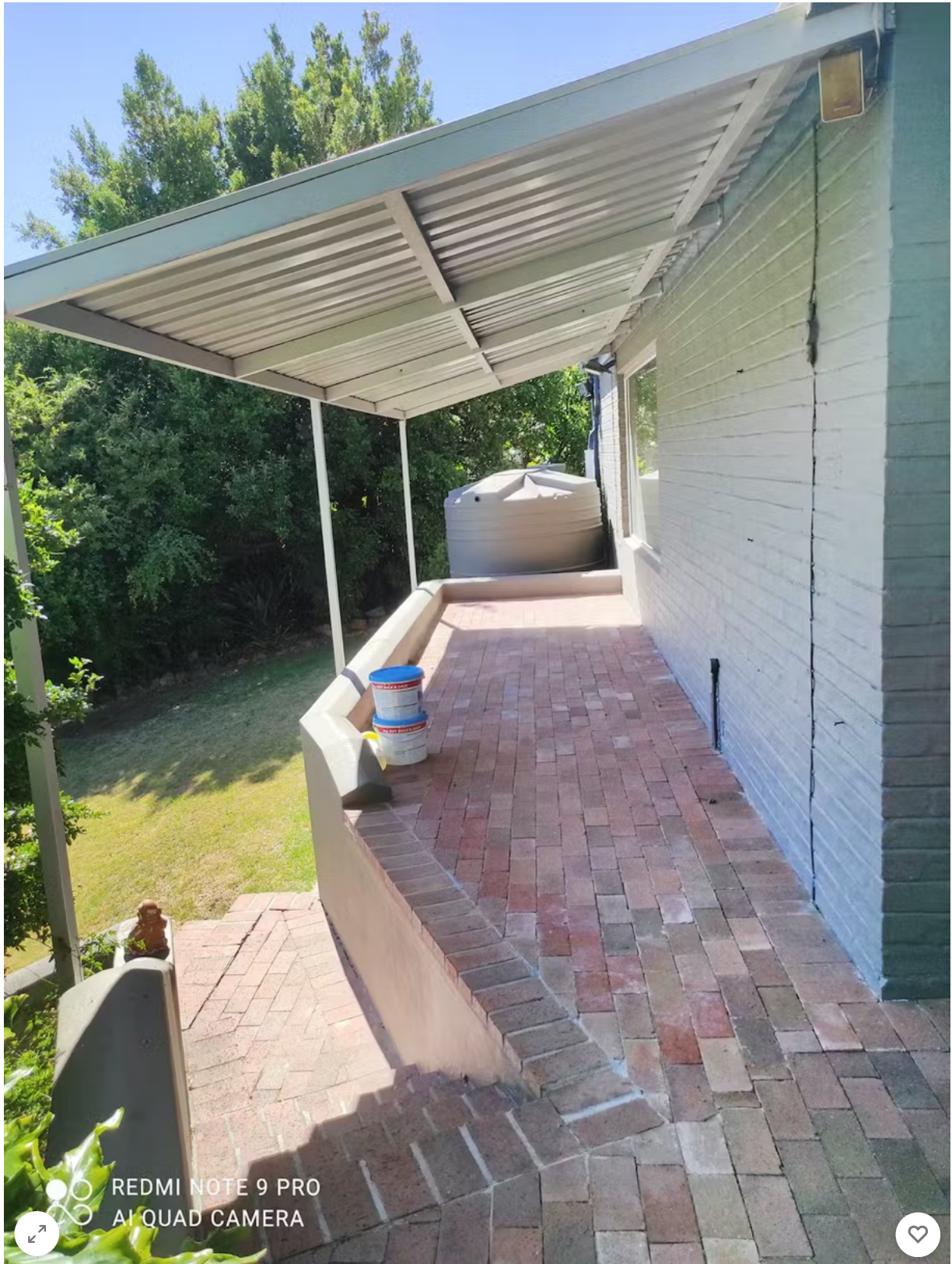
Before: A walkway in brick wasn't very functional.
