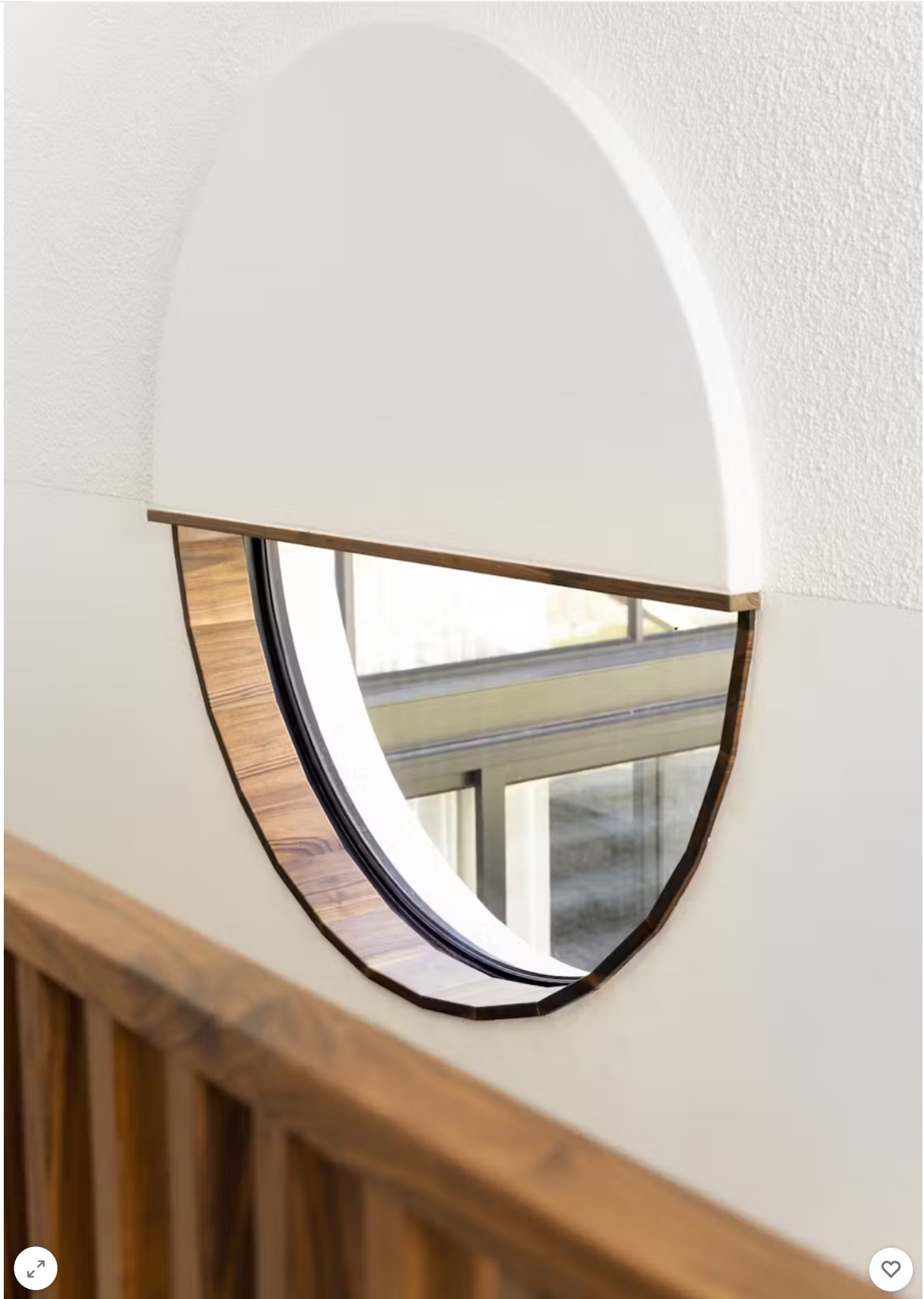
A half-moon window trimmed in walnut at the top of the stairs provides visual interest and natural light.
